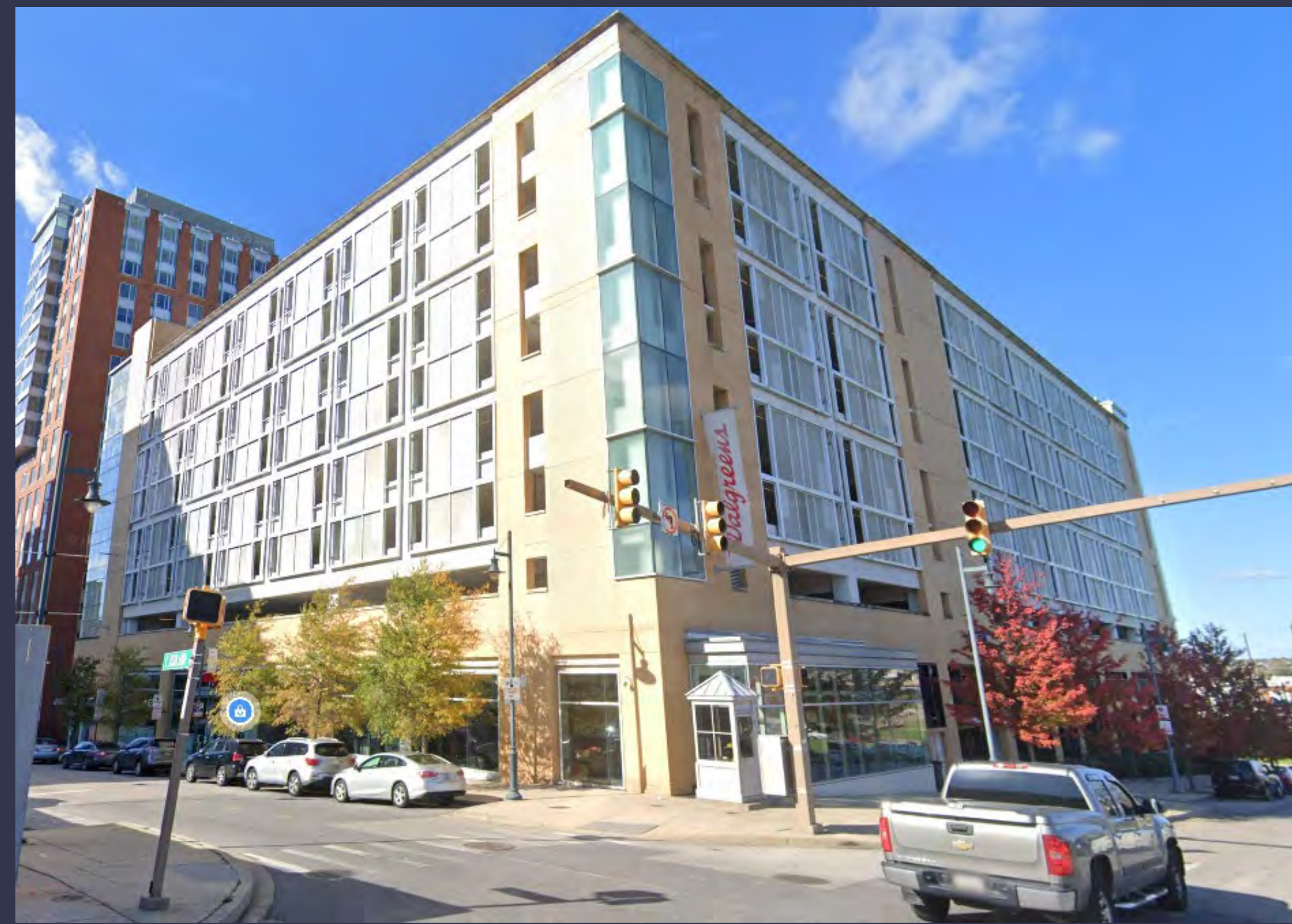
Ashland Avenue Parking Garage with ground floor Walgreens – Baltimore Source: Google Earth
