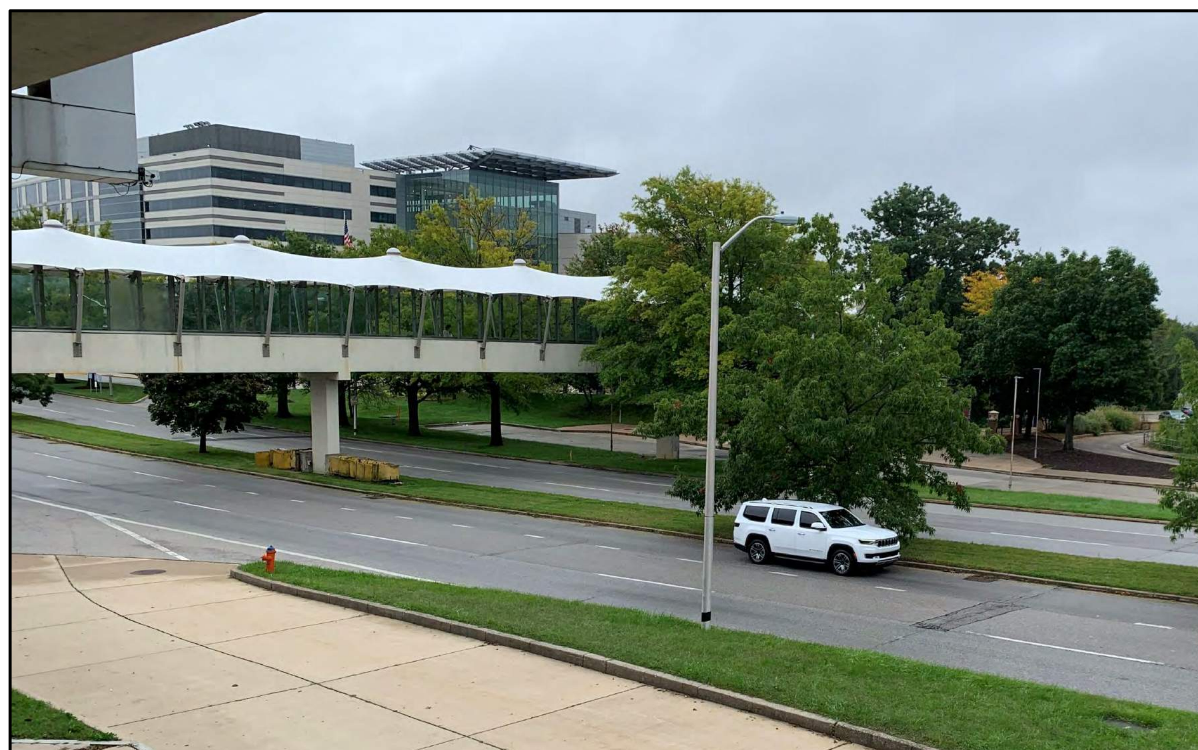
Existing Access to Station
