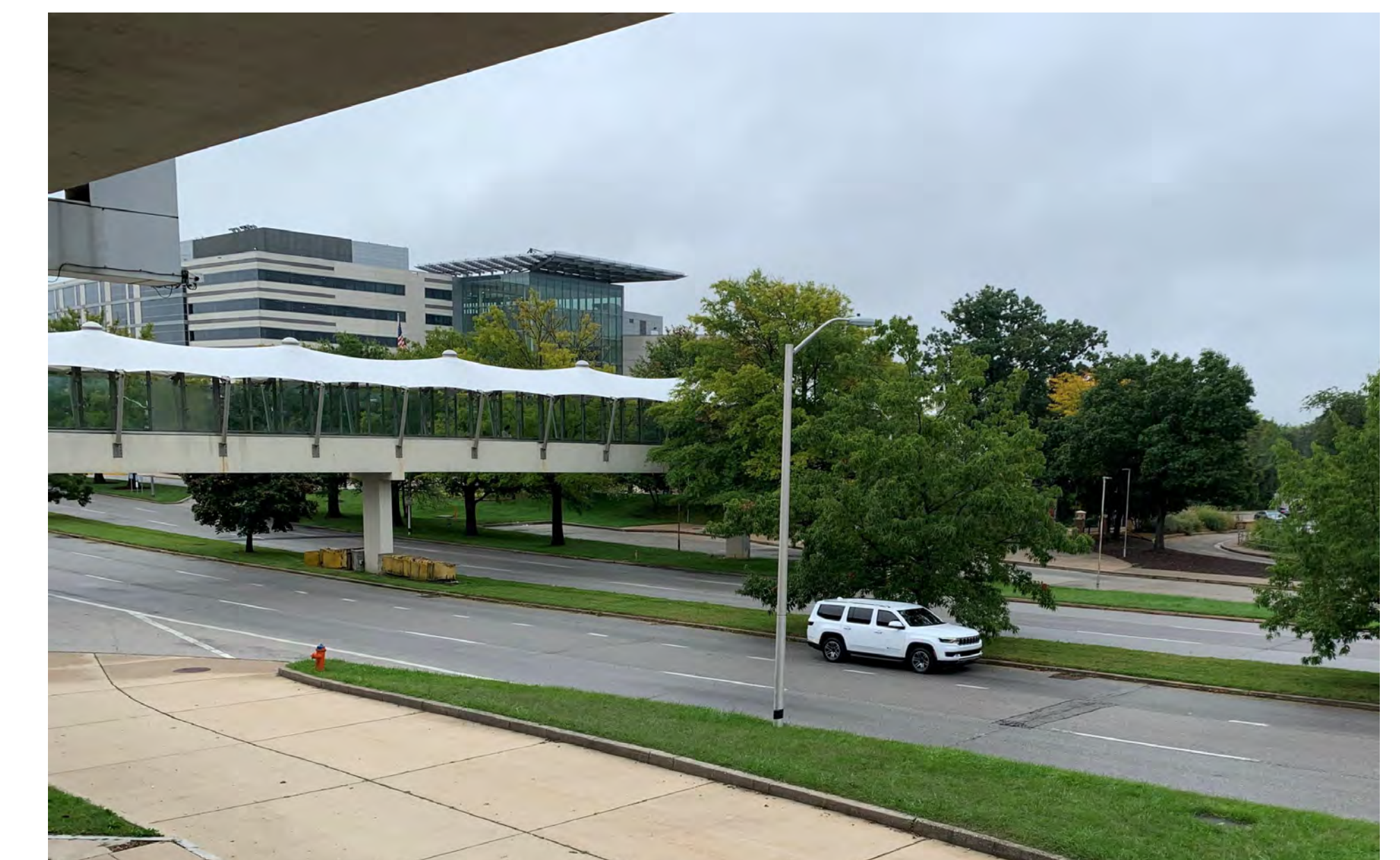
Existing pedestrian bridge connecting to the station (looking west)
