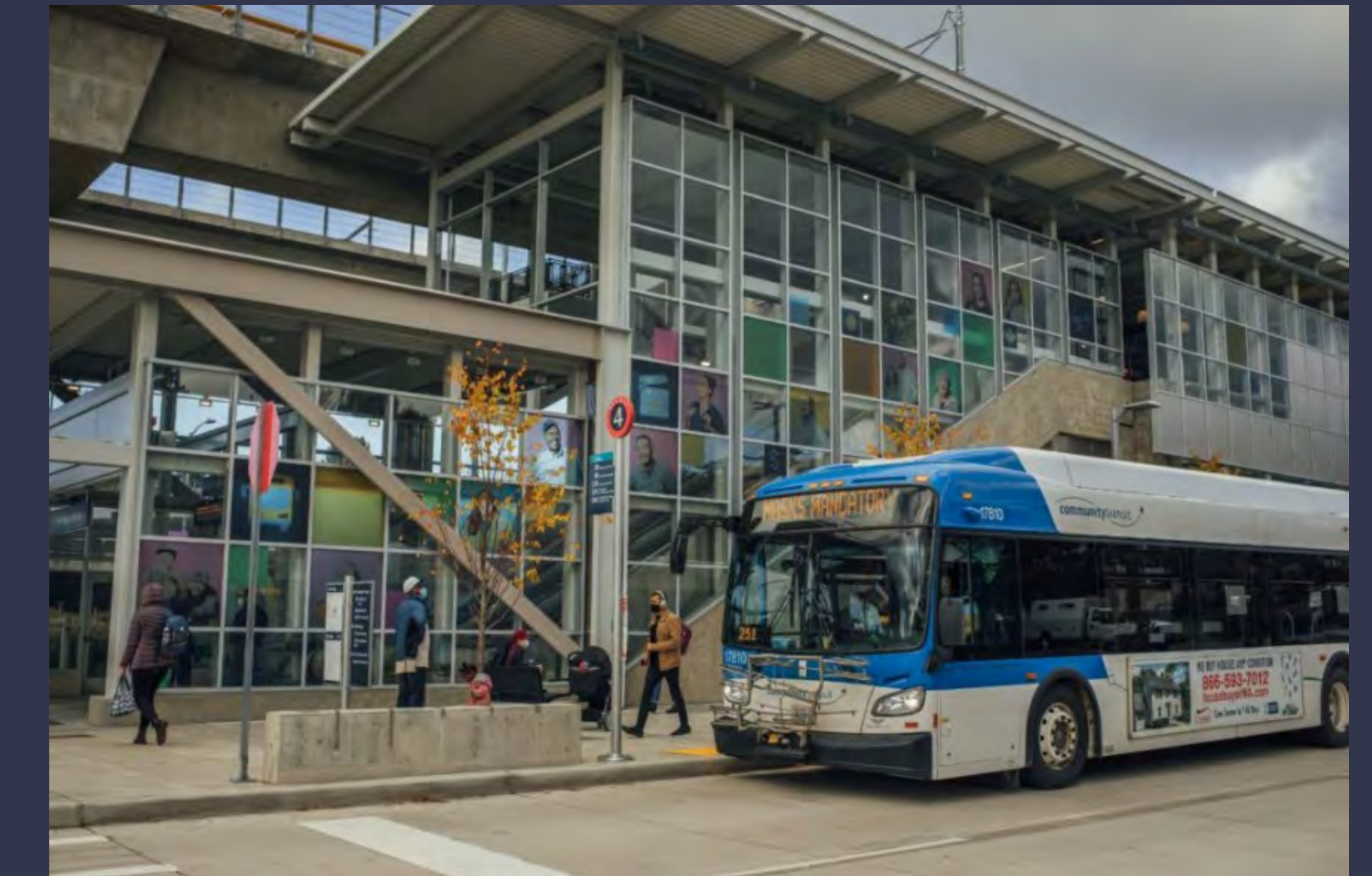
Snohomish County, WA Light Rail Station Source: Community Transit
