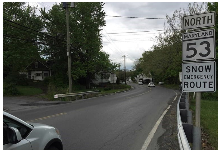
Figure 4: A stretch of US 220 in the Project area with no safe sidewalks for pedestrians.
