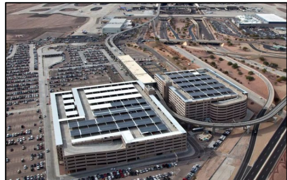
Rooftop solar parking canopies at PHX
