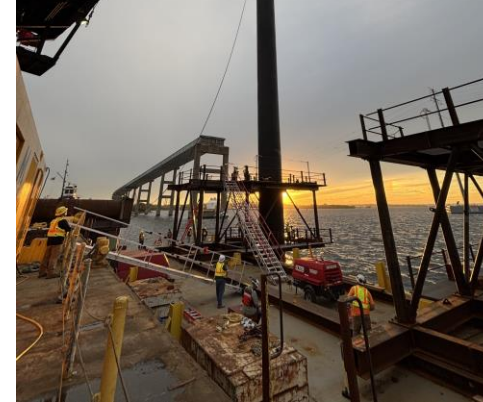
Test Pile machinery on flotilla during sunset
