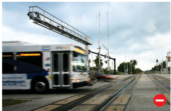
Whenever possible, transit modes should be routed, and their stops situated, to minimize conflict with one another. The example above with a bus crossing multiple train tracks to access the train station should be avoided if it is possible to have the bus and train routes run parallel. Source: KAI
