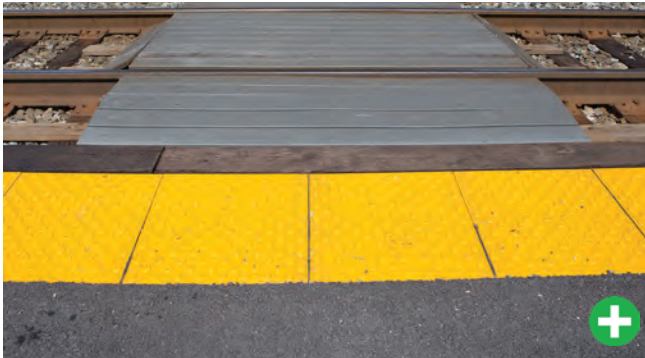
Detectable warning strips are used to alert passengers of a track crossing. Source: KAI
