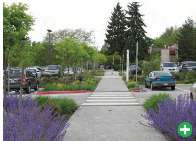
This parking lot utilizes code-required landscaping for bioswales and other innovative stormwater collection mechanisms while also providing a central sidewalk with signage and wayfinding. Source: SvR Design
