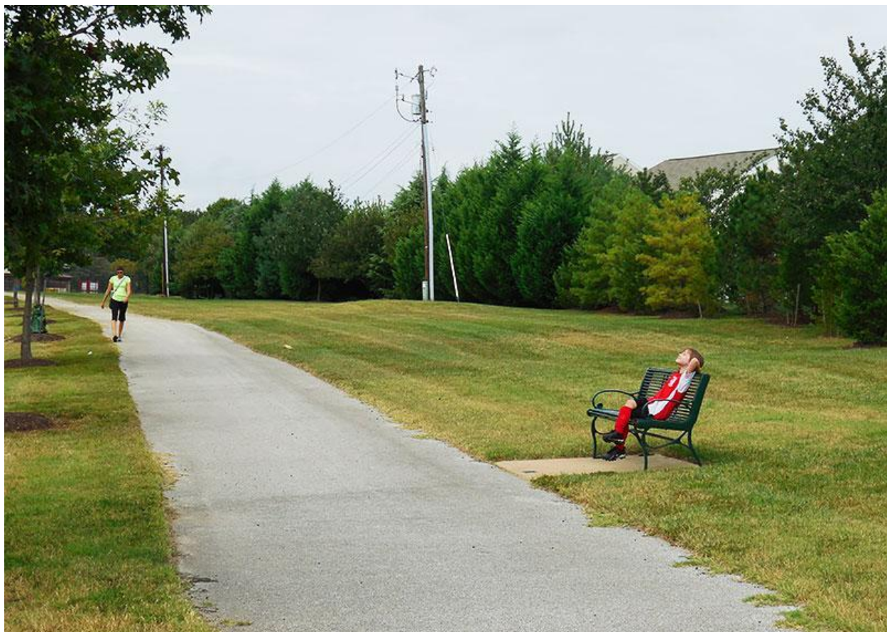
Anne Arundel County completed Phase 1B of the Broadneck Peninsula Trail in 2024. Image source: aacounty.org .
