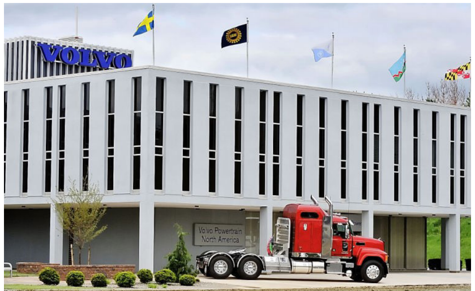
The Volvo Powertrain factory in Hagerstown, MD, covers 1.5 million square feet of floor space and employs about 1,700 people
