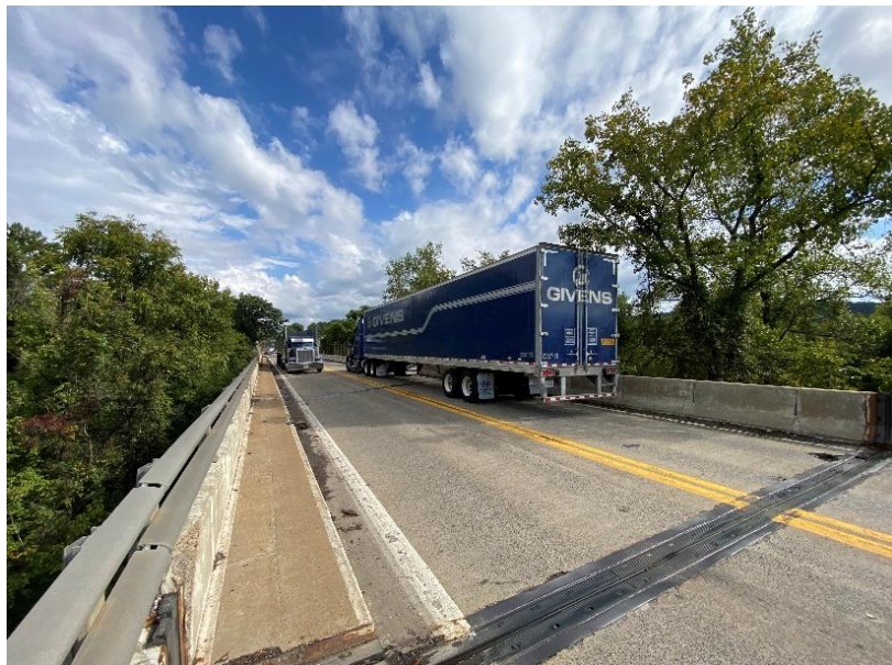
Figure 10 Trucks Navigating the Tight Two-Lane Cross Section on the US 522 Bridge 210043001
