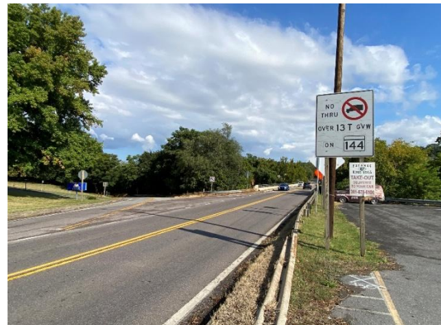
Figure 13 Access to the US 522 Bridge 210124001 with a Weight and Size Restriction Signage for Heavy Trucks
