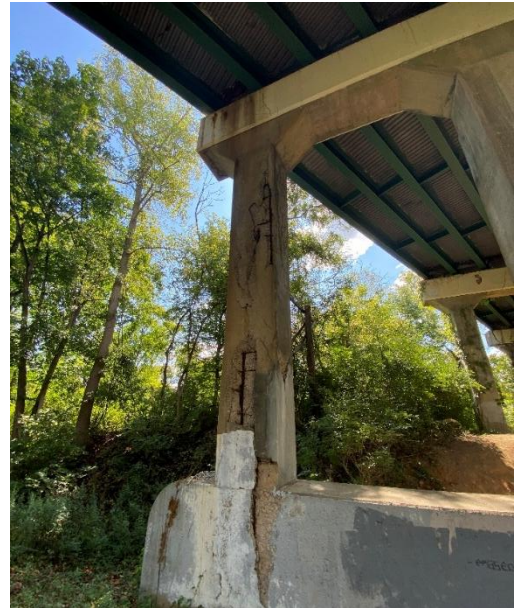
Figure 1 Deteriorated Column and Exposed Girders on the US 522 Bridge 210043001
