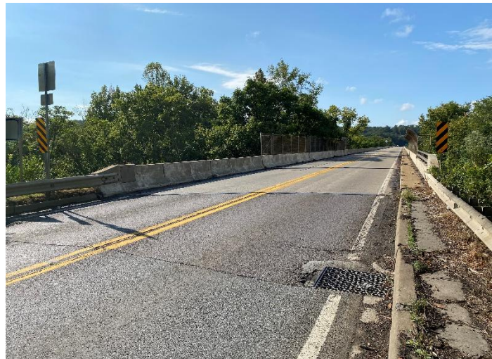
Figure 7 Elevation View of the US 522 Bridge 210043001
