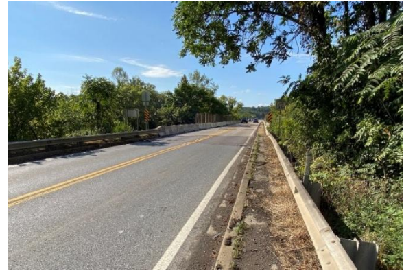
Figure 4 US 522 Bridge 210043001 Runs Over The Potomac River between MD and WV
