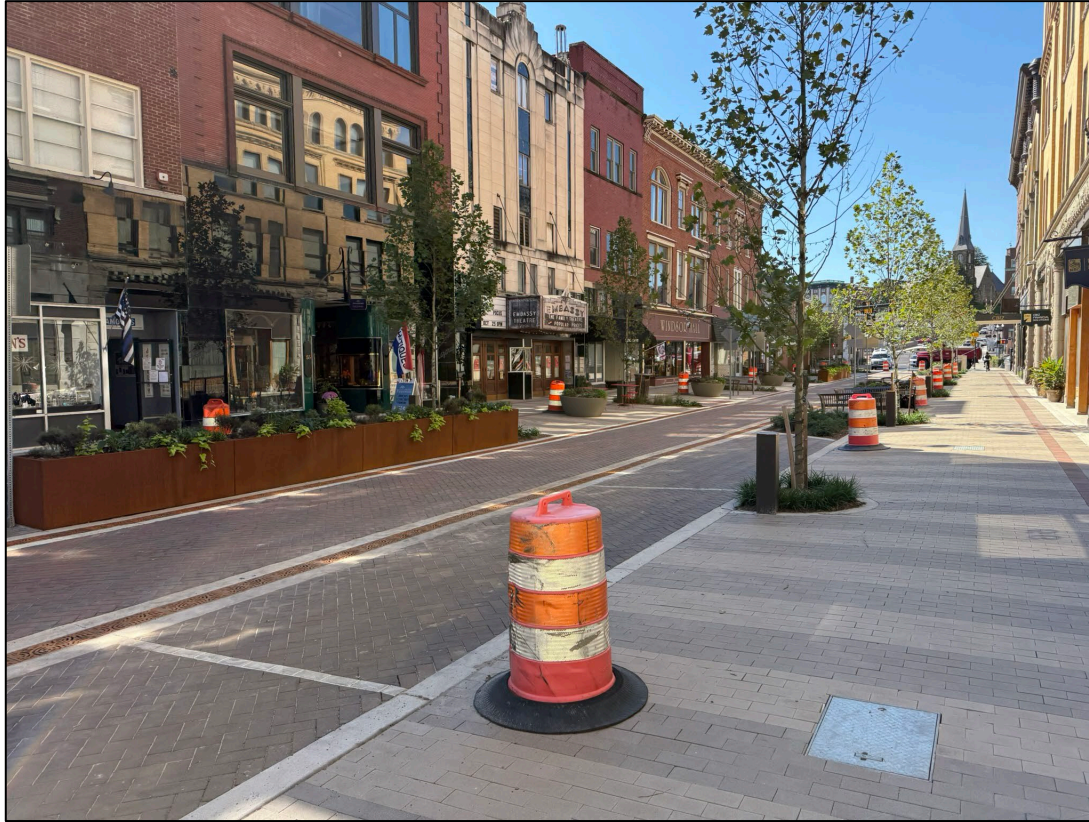
Baltimore Street Access - City of Cumberland
