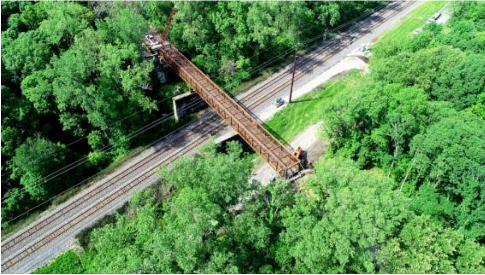
Figure 14. MCT Goshen Trail Bridge Over Active Railroad Tracks
