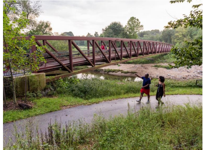
Figure 6: Herring Run Trail Bridge in Baltimore
