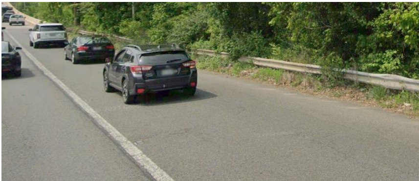
Figure 5. Current Bridge Approach Shoulder Width
