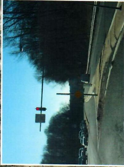
There is currently a single left turn lane from southbound US 1 onto MD 24 at this half signalized intersection which backs up into the high speed southbound through lane. In lieu of the full interchange currently proposed for the long term improvement, Harford County proposes that MDOT program funding to design and construct a second left turn lane onto MD 24 from US 1 Bypass to increase capacity and eliminate this very hazardous condition. This improvement is the County's number one priority.
