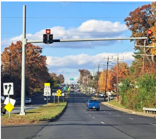
The MD 650 corridor between MD 193 (University Boulevard) and Powder Mill Road is planned for safety improvements as part of the Maryland State Highway Administration's Pedestrian Safety Action Plan
